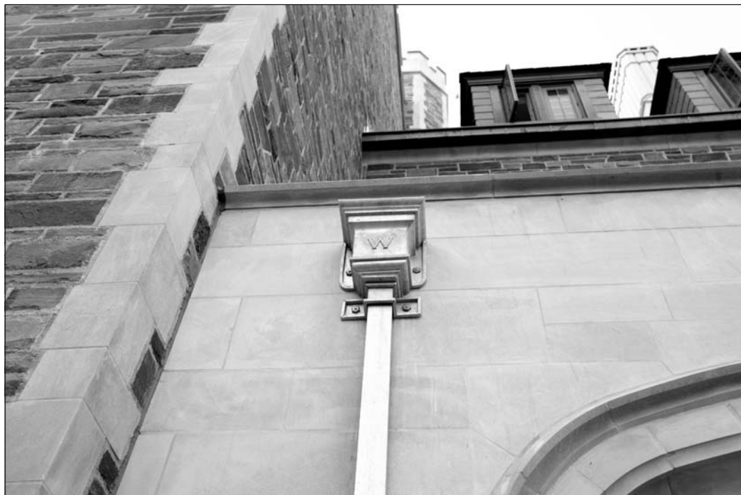
All in the details. Roof and exterior work at Princeton University's Whitman College completed by the Bregenzer Brothers firm included hand-cut hexagonal brass anchor-bolts, above, for the copper drainage system they installed throughout the college, including over 80 hand-fabricated copper leader heads like the one at left.
